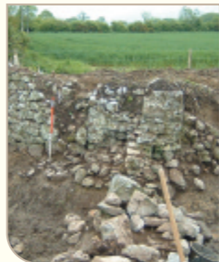
Mortar-bonded townland boundary wall at George's-Land .
